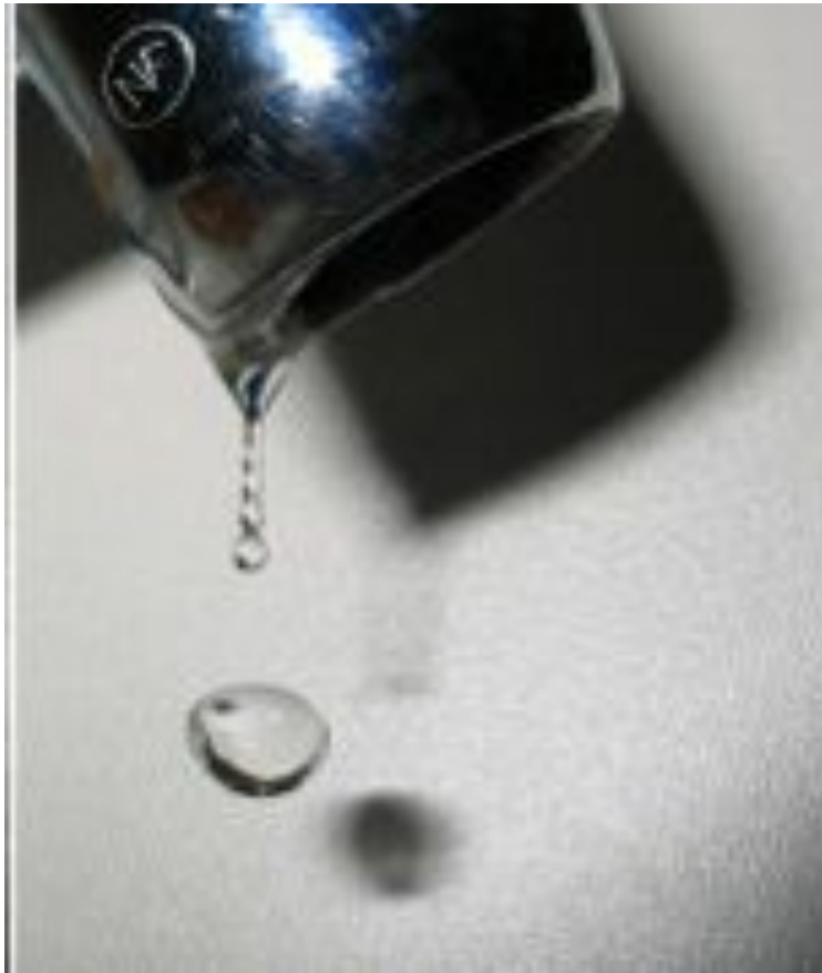
Figure 18.18: One drop per second from a dripping faucet wastes 2,700 gallons of water per year and adds to sewer and/or septic costs, as well.
